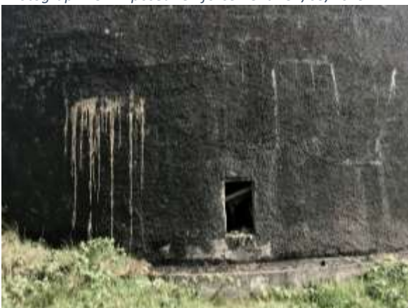
Photograph 15 - Ventilation opening to south - 31/05/2019
