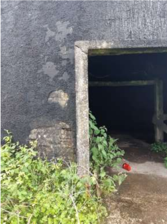
Photograph 7 - Rendered entrance door surround - 31/05/2019
