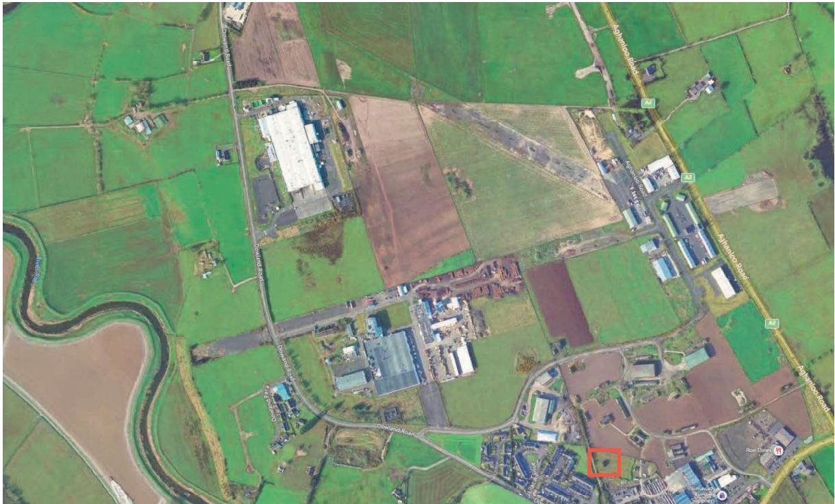
Image 13 - Location of RAF Trainer Gunner Dome in the former Limavady Airfield (extract from Bing maps)
