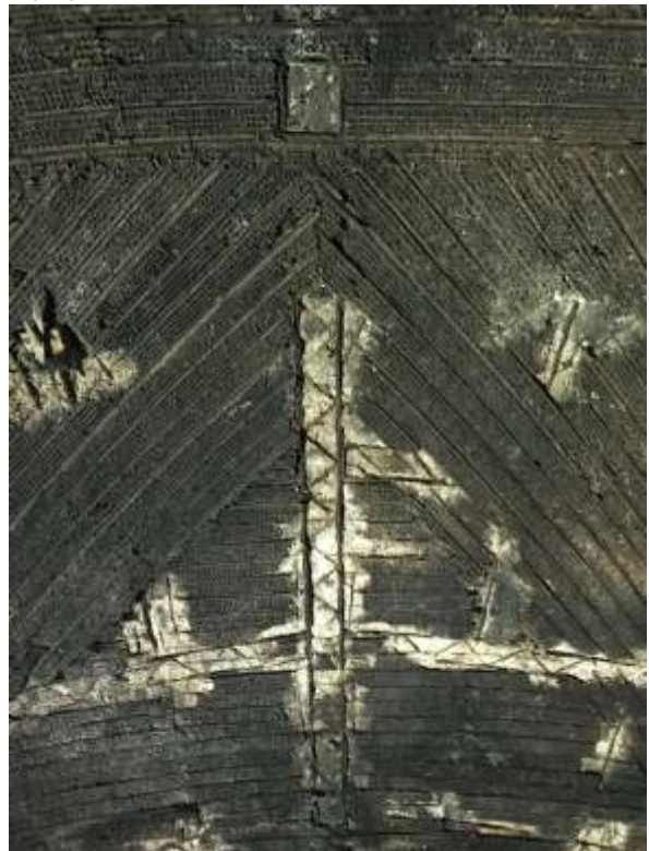
Photograph 14 - Exposed reinforcement - 31/05/2019
