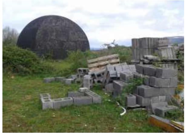
Photograph 2 - Poor setting from south - 31/05/2019
