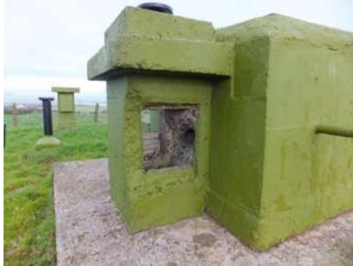
20 Cold War Era Royal Observer Corp Bunker (Nuclear Shelter) Cranagh Road
