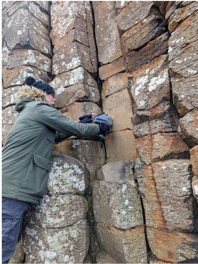
Fig 8. Handheld XRF Grid Survey of block/joint panel surrounds
