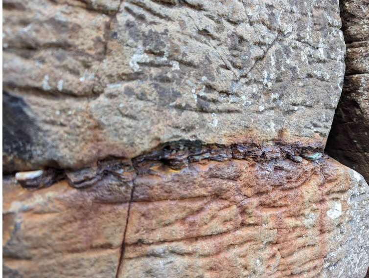
Fig 4 Substantial evidence of coin jointing deposition, oxidation of coin deposits and brown surface staining originating from the coin mass (Test survey 'panel').
