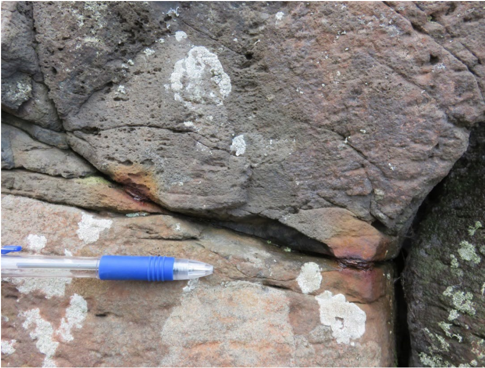
Image 5. Image showing a fragmented joint margin resulting from the expansive delamination of coins inserted into the joint. Note the missing piece of basalt rock above and to the right of the pen tip; residual pieces of two coins can be seen in the joint recess. The pen, for scale, has a diameter of 10 mm at its widest point.
