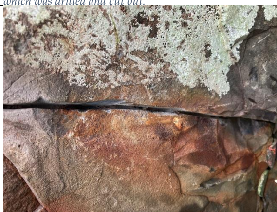
Figure 6 – Area 1 – Detail showing abrasion on the stone from battery powered rotary tool
