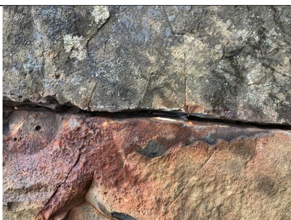
Figure 5 – Area 1 – Detail showing slight abrasion on the stone from battery powered rotary tool
