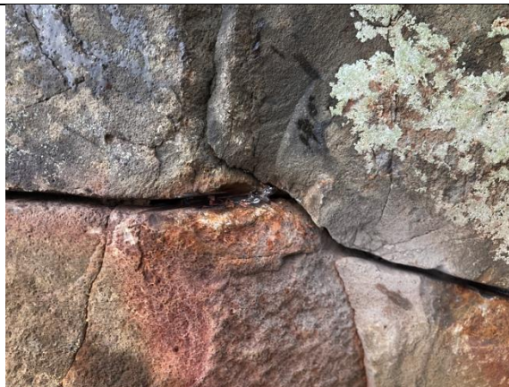
Figure 4 – Area 1 – Detail showing compacted metal, which was drilled and cut out.
